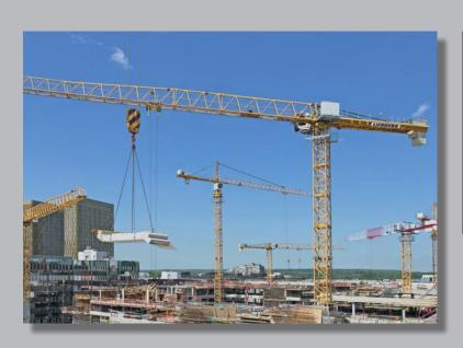
**Challenge:** Numerous joints need to be bolted together during the erection of a tower crane. The stability of the tower crane is dependent on the integrity of its bolted sections. The precise application of torque is critical to ensure the tower crane's stability.
